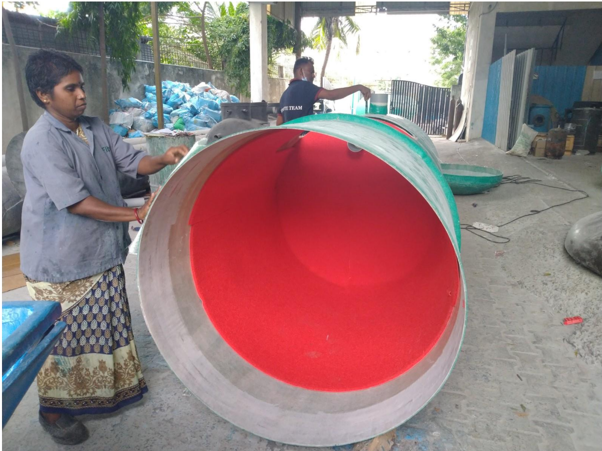
Assembling of 4 KL Bio-septic tank
